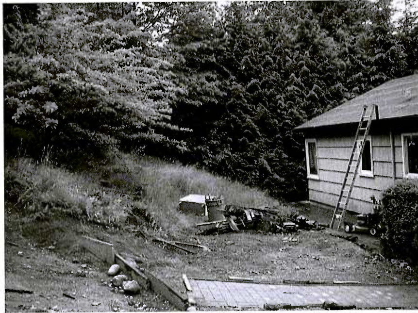
Figure 6. View east at north side of house at 3715 Dollarton Highway.
