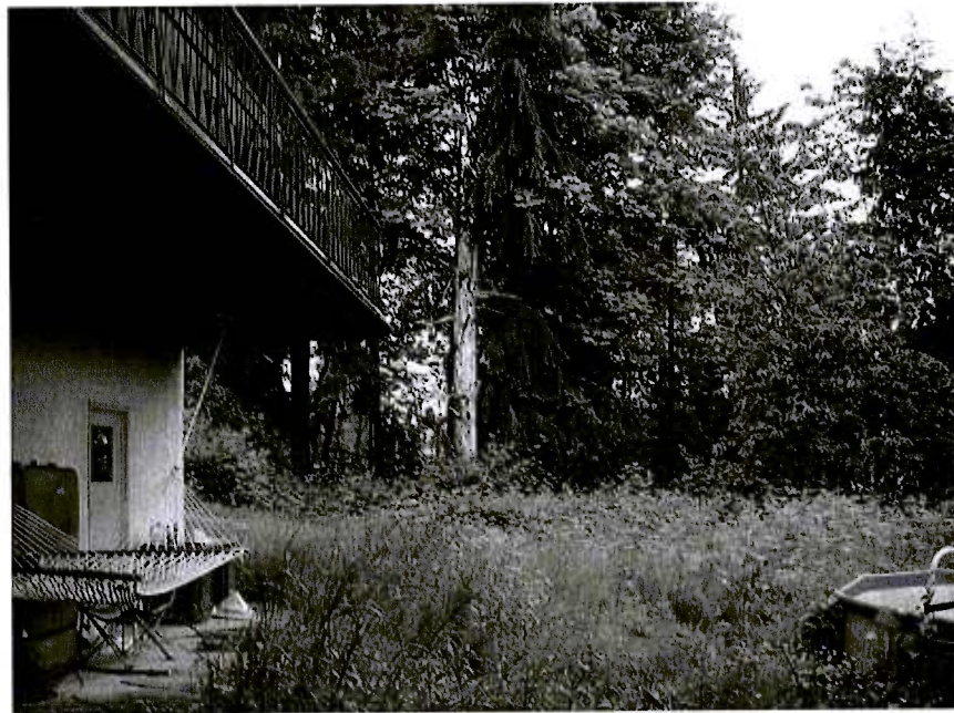
Figure 7. View east at south side of house at 3739 Dollarton Highway.
